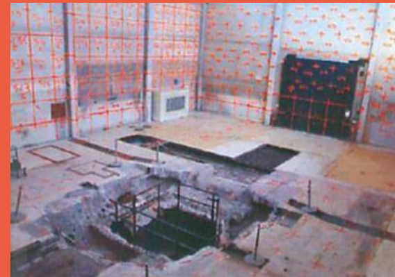
Complete mapping of the concrete structures
