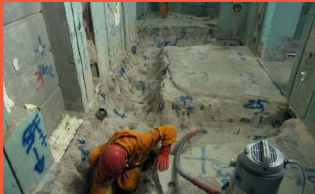
Removal of deep contamination
