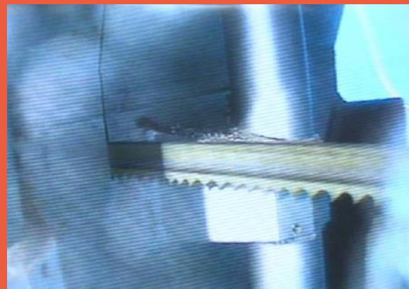
Dismantling the internal parts with band saw at Stade nuclear power station, Germany
